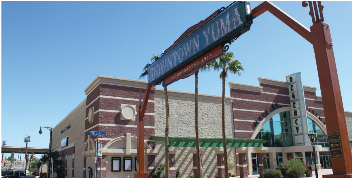
Downtown Yuma – As jobs increase in the region, roadway improvement will be needed to support growth. (Source: Kimley-Horn)
